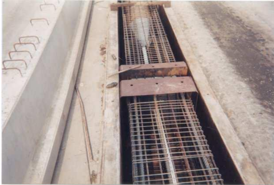
30" sq. Sure-Lock Splice – Male & Female parts in casting bed, splice anchor rebar screwed into splice plates inside spiral.
