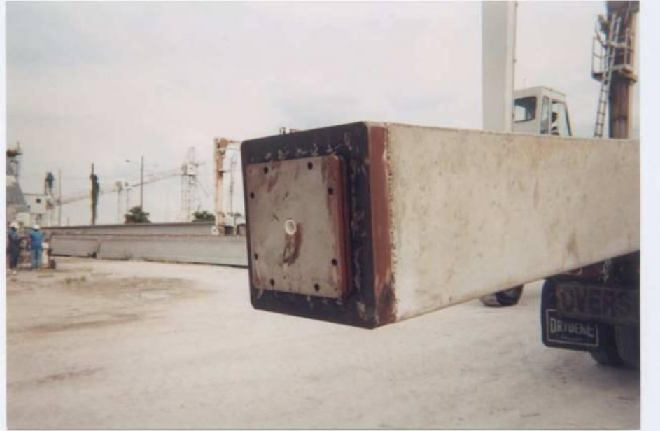
30" sq. Sure-Lock Splice – Top pile segment with Male main plate Splices were for FDOT bridge project
