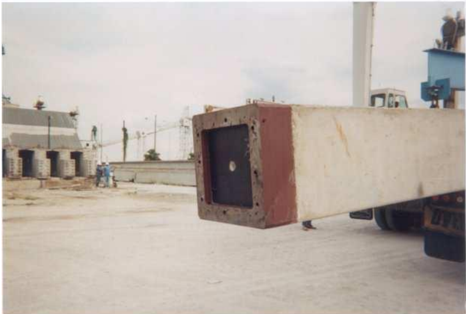
Bottom Pile Segment – with Female Splice end, showing recess for square Male Plate.
