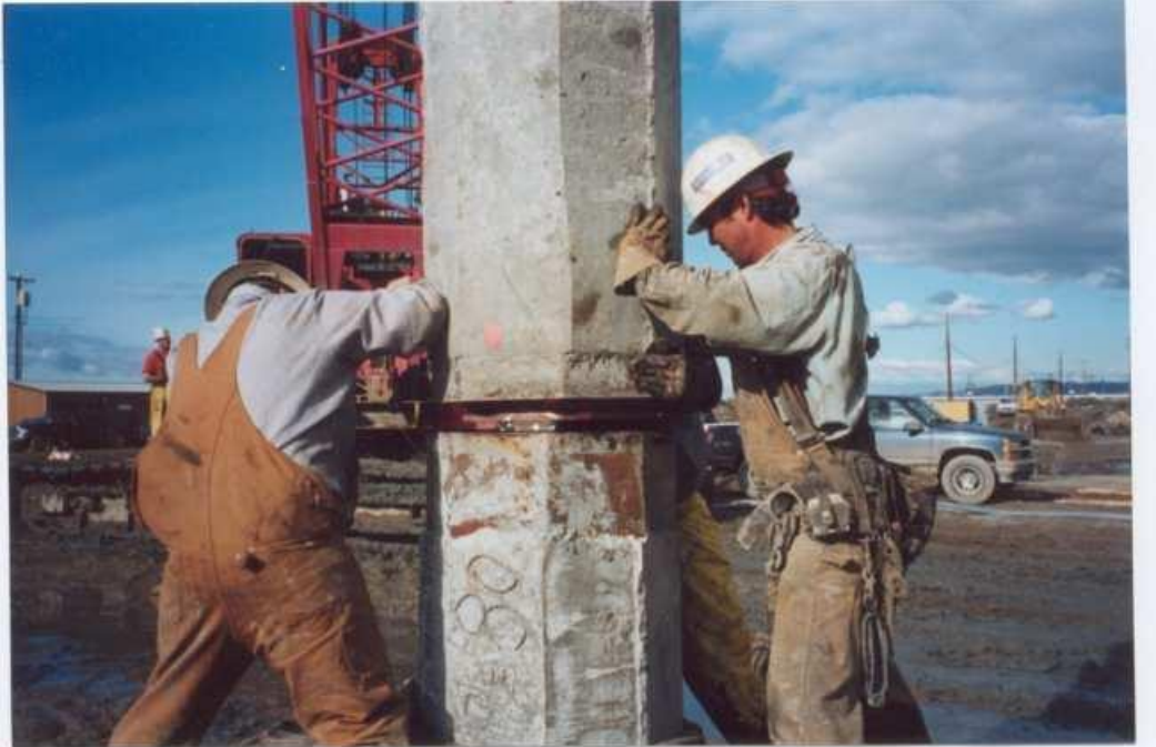
24" oct. Sure-Lock Pile Splice – inserting the top segment Male into bottom segment Female splice half.
