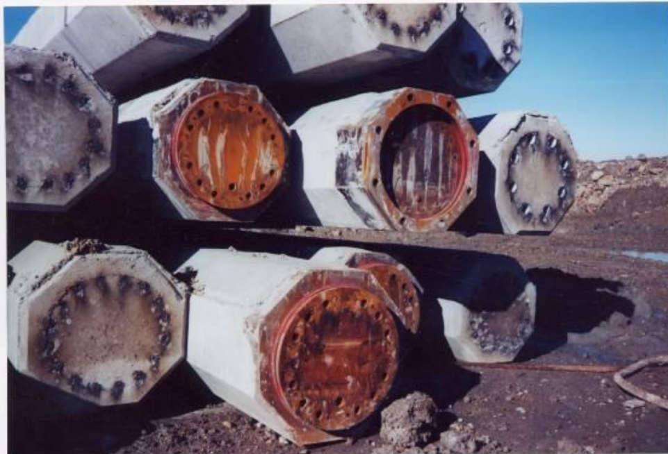
24" oct. pile, Male and Female splice ends on 80 ft. pile segments
