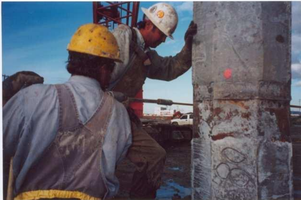
Driving one of the two locking bars into the grooves of the Male & Female plates with an air hammer to form a circular shear key.
