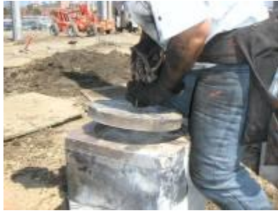
Removing the Drive Plate
