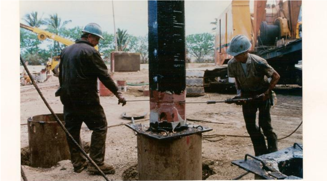
5000 – 16" octagonal splices for Honolulu Keehi Interchange. 3 – 90 ft. segments per 270 ft. long pile with 3" center tube for verification of pile integrity.
