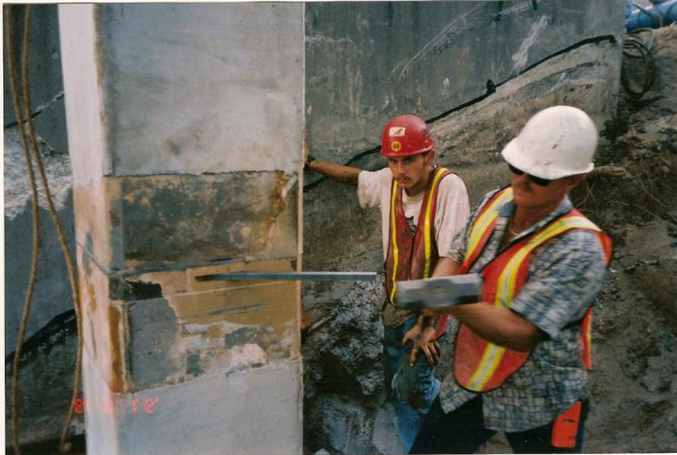
18" sq. Splice for FDOT bridge – After mating the splice halves, 2 high-strength steel locking bars are driven into the matching Male and Female splice grooves with sledge or Rivetbuster.
